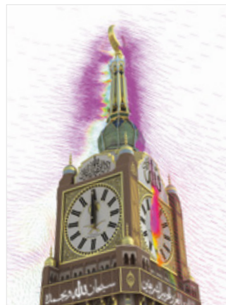
Fig. 5: CFD wind simulation results with velocity vector time snapshot in a vertical section.
