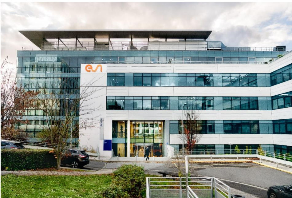
ESI Group Headquarters Rungis, France.
